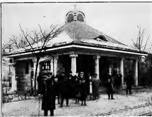
SLIDE No. 36.—COMBINED TELEPHONE KIOSK, TRAM WAITING ROOMS AND CONVENIENCE.
